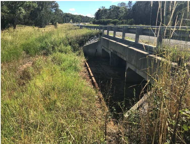
Plate 1 Three Cell Culvert System Beneath Ocean Drive
